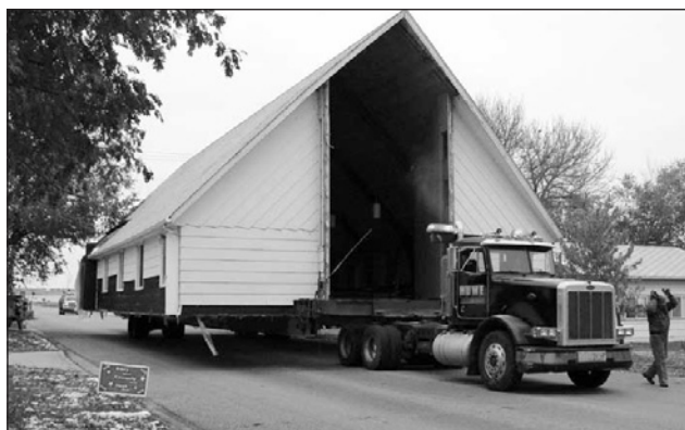
Trinity Free Lutheran Church, Minnewaukan, N.D., was moved Oct. 24. The church was in a low spot that was in danger of flooding from the waters of nearby Devils Lake. In fact, the heating ducts in the concrete foundation had flooded, so a settlement was made with the National Flood Insurance Program, which provided funds so the church could be moved. There was no room for other vehicles on US 281 through Minnewaukan. The church is now situated on Main Street.
